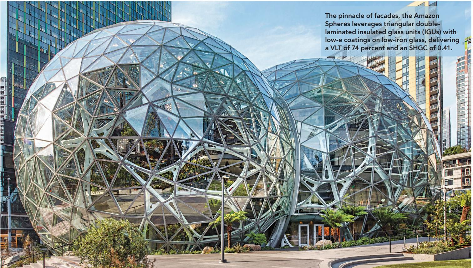
The pinnacle of facades, the Amazon Spheres leverages triangular double-laminated insulated glass units (IGUs) with low-e coatings on low-iron glass, delivering a VLT of 74 percent and an SHGC of 0.41.
